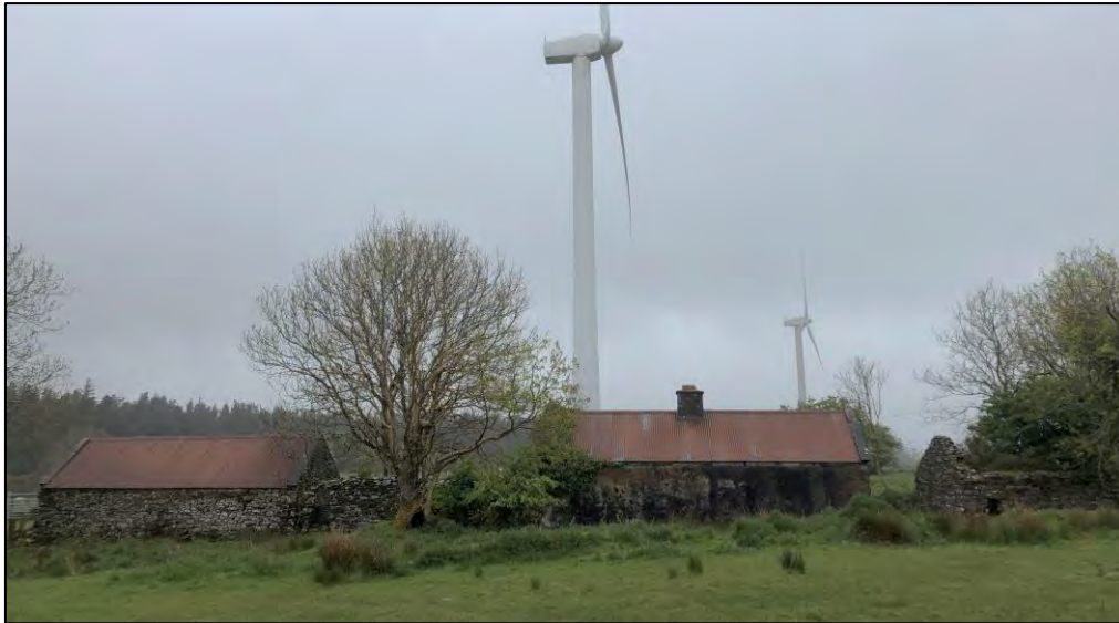
Plate 4-2 Three derelict structures within EIAR study area - South facing elevation
