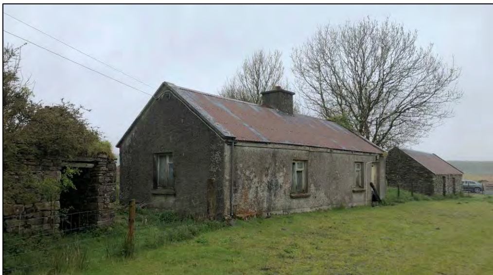
Plate 4-1 Three derelict structures within EIAR study area - North facing elevation
